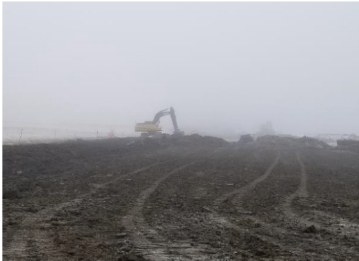
Levelling off ROW and clean up – km 221+920 – Nov 30, 2018
