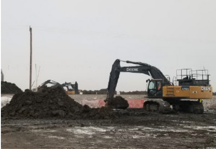
Digging bore pit – km 265+160 – Nov 29, 2018
