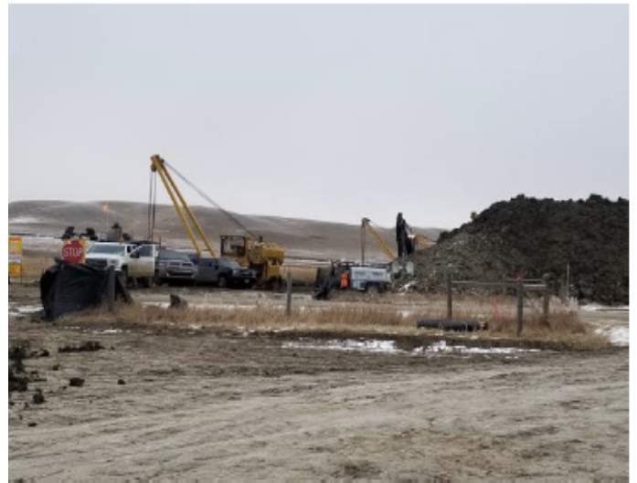
Tie-in at heritage site - km 221+890 – Nov 26, 2018
