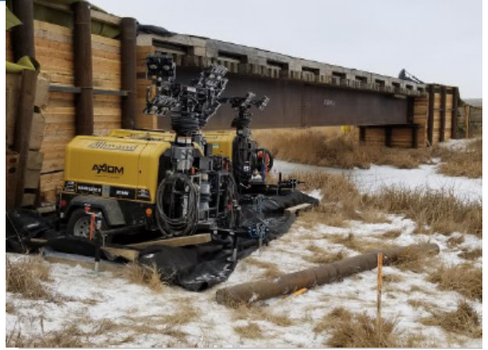
Containment for plants – km 255+150 - Nov 28, 2018
