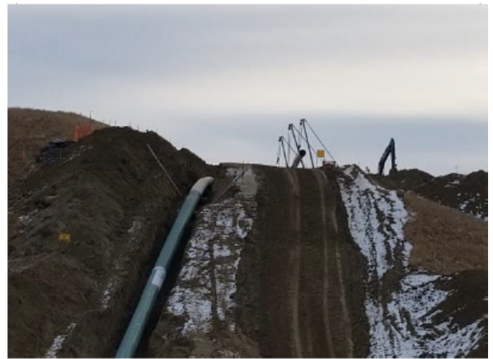
Lower in tie-in section – km 222+600 - Nov 27, 2018
