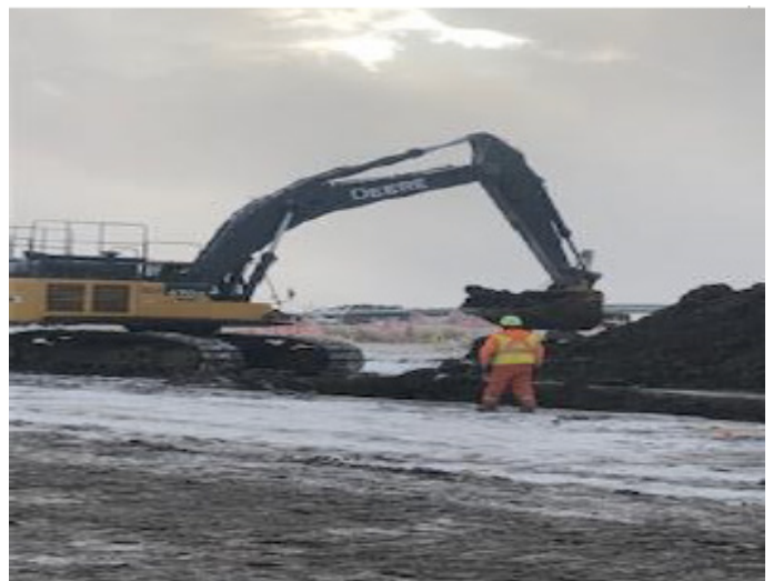
Digging ditch for tie-in – km 227+900– Nov 29, 2018
