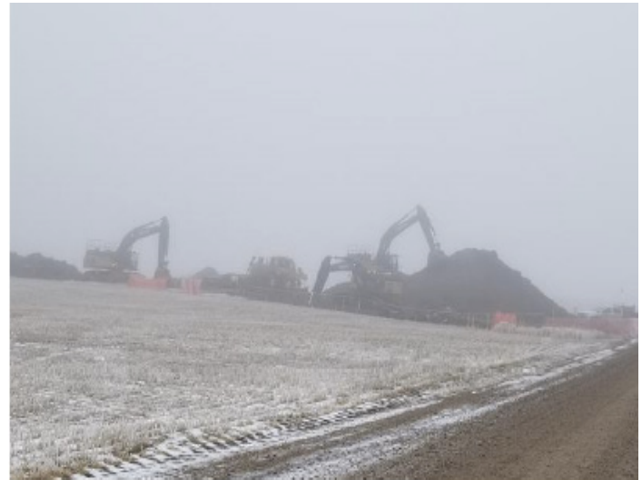
Digging tie-in section – km 262+631 – Nov 30, 2018
