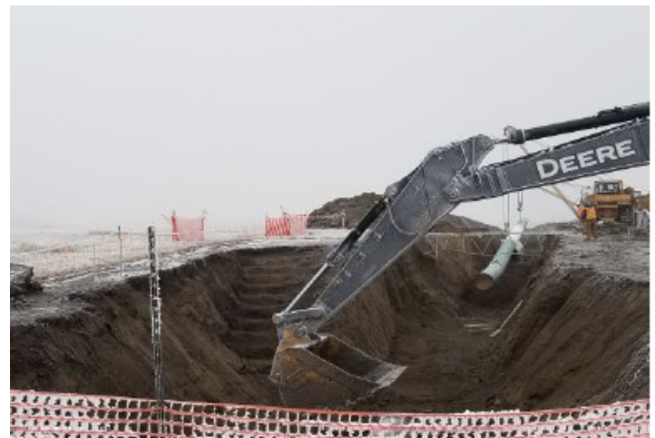
Lower in tie-in section under hotline – km 262+640– Dec 1, 2018
