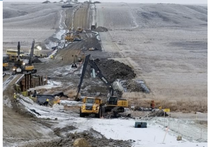
Loading ice and installing aqua dam –km 255+300– Nov 29, 2018
