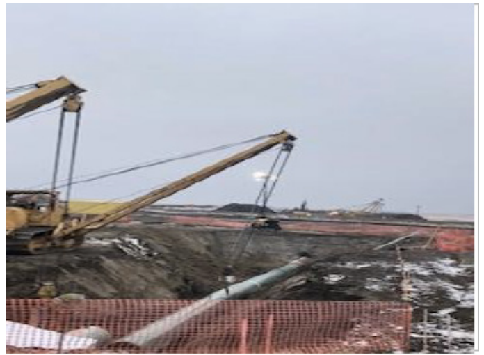
Lining up the cut – SF 170 – Nov 28, 2018
