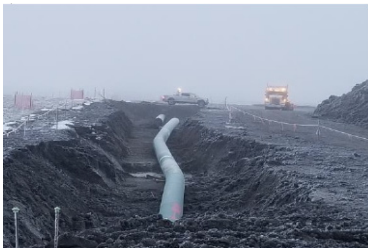
End tie-in – km 266+760 – Dec 1, 2018
