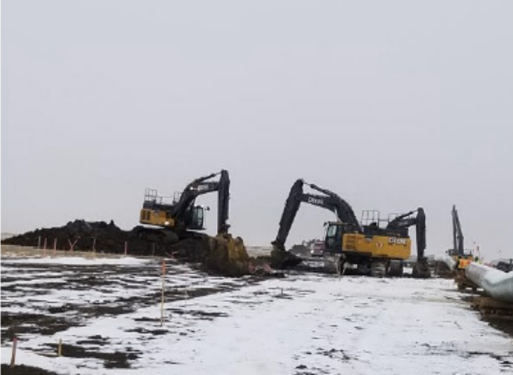
Digging tie-in section - km 221+185 – Nov 26, 2018
