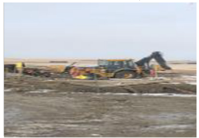
Rubber tire hoe working – km 195+500 – Nov 27, 2018
