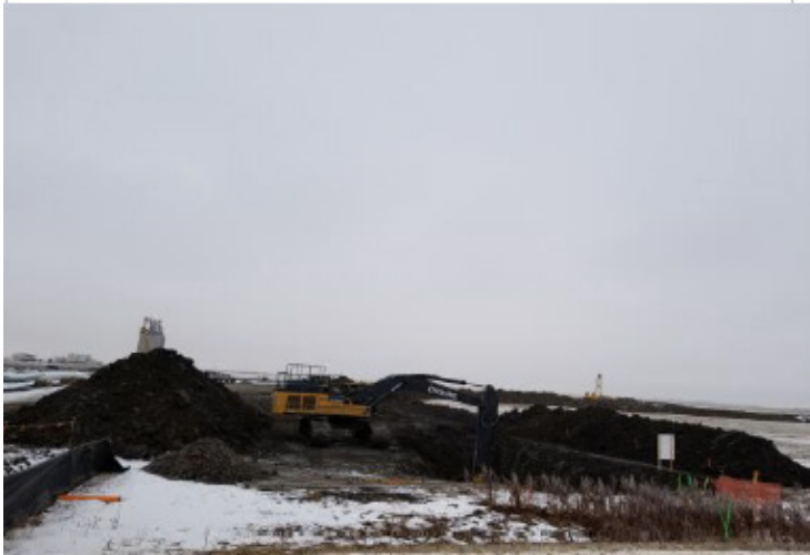
Digging bore pit – km 265+060 – Nov 28, 2018
