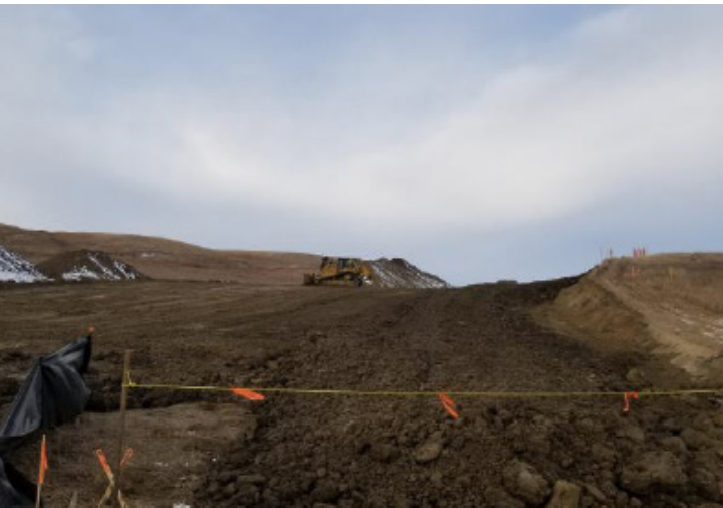
Levelling the ROW – km 222+670 – Nov 27, 2018
