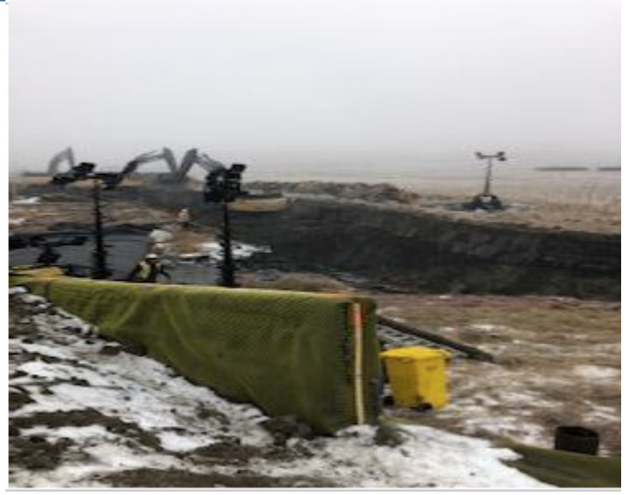
Excavator digging mainline ditch – SF 162 – Dec 1, 2018
