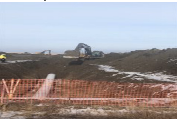
Excavator shading tie-in – km 232+800 – Nov 27, 2018
