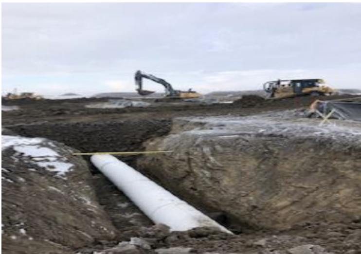
Dozer and excavator levelling ROW – km 223+600 – Nov 29, 2018
