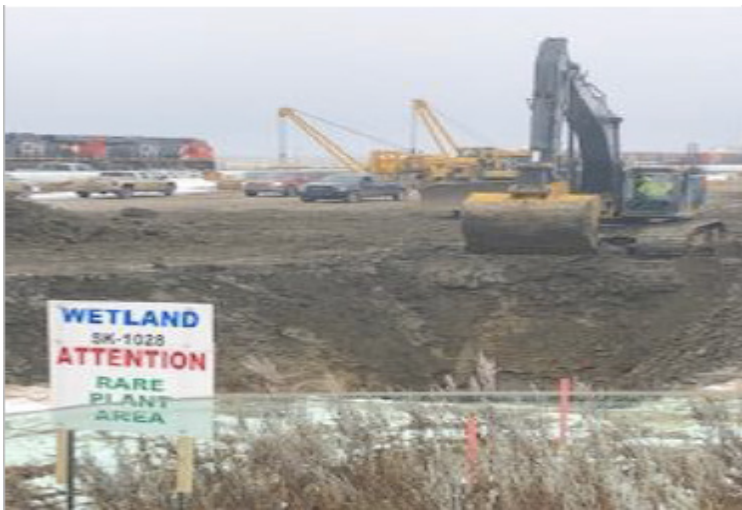
Excavator digging bell hole through rare plant area – SF 169 – Nov 28, 2018
